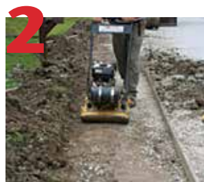
Spread fill/bedding layer evenly, compact well.
