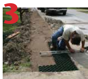
Spread sand over the bedding layer, compact well. Position GrassGrid and ensure everything is level.
