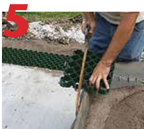
GrassGrid is easily cut using a hacksaw.
