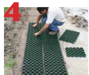
Continue to lay GrassGrid. Click parts together and stagger joints. Use anchor nails on perimeter grids (2 per grid). For extra security (especially on slopes) use additional nails on interior grids where desired.
