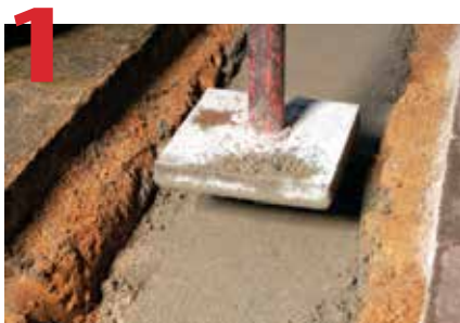
1 Excavate area to accommodate trench drain and 4" concrete surround, compact base.
