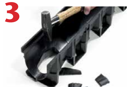
3 Knockout channel base for outlet at required position.
