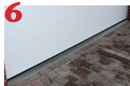
Clean away debris, remove protective plastic.
