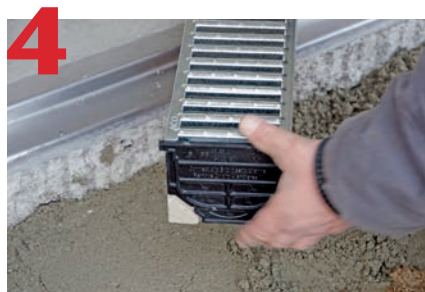
Fit end caps. Insert grates. To keep concrete from getting onto grates or seam, protect grates with plastic.
