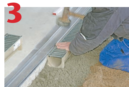
Lay channels starting at outlet. Set a string line at required height to ensure level. Seal joints if required.
